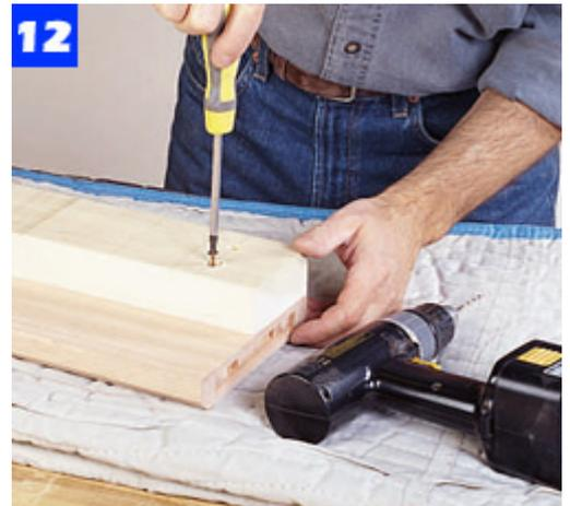
Locate the support-rail ends 1/16 in. short of the main rail ends. Then, screw the poplar support rails in place.
